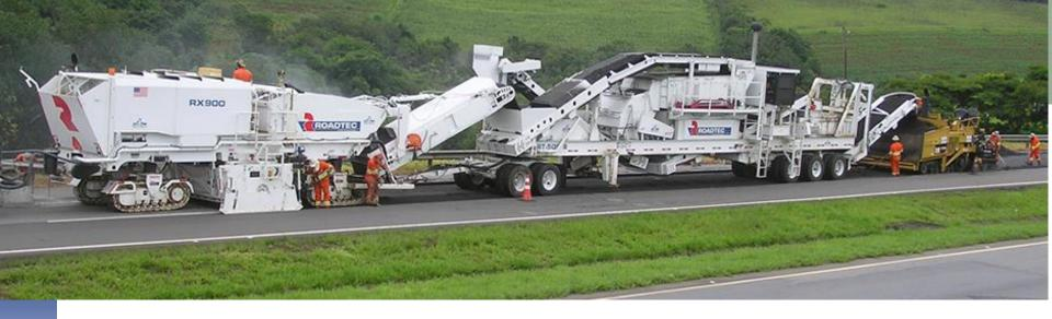
In Peru, cold in-place recycling (emulsion-based) has been used for over 20 years to solve numerous pavement distresses in a cost-effective manner.
